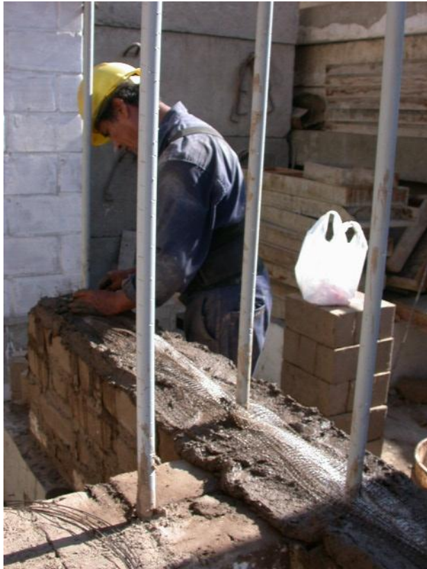
Internal PVC pipes and plastic mesh reinforcement
