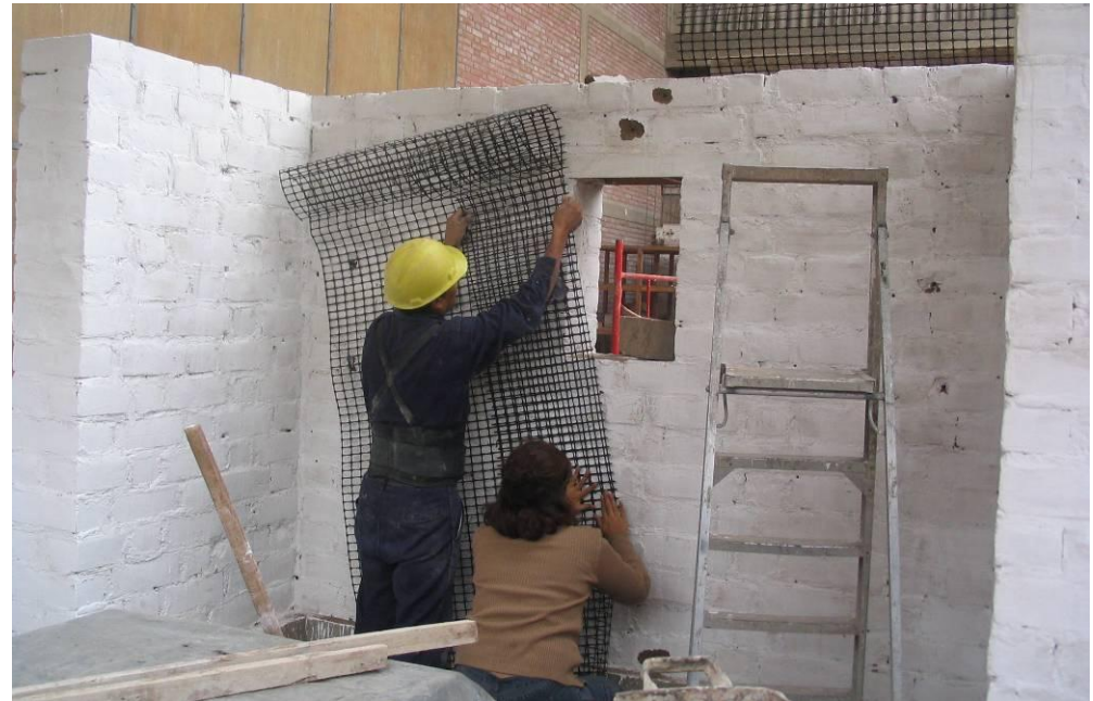
External geomesh reinforcement
