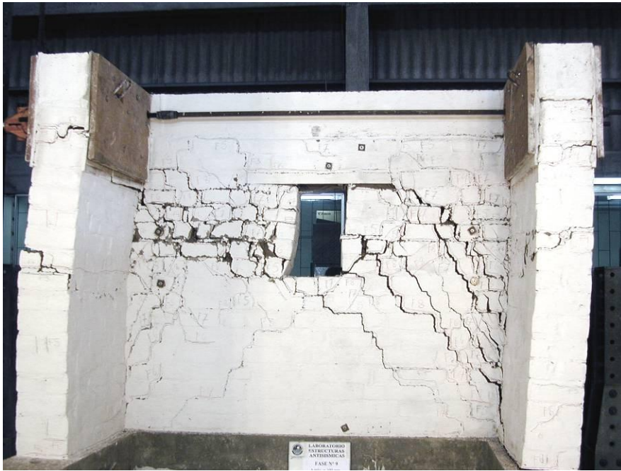
Internal reinforcement: a net of PVC tubes and plastic mesh
