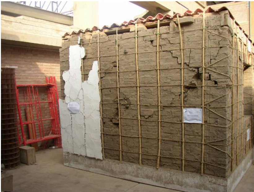
External reinforcement net made with cane rods and rope
