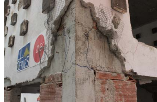
RC cracking (mid-height and joint)
