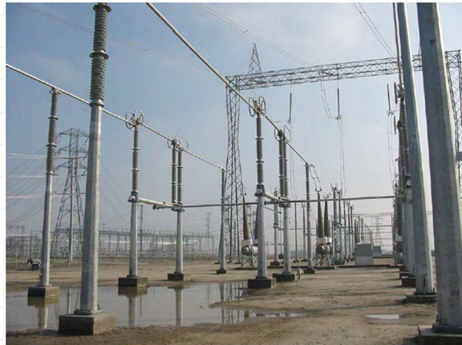
Typical field installation of vertical-break 500-kV disconnect 3-phase switch
