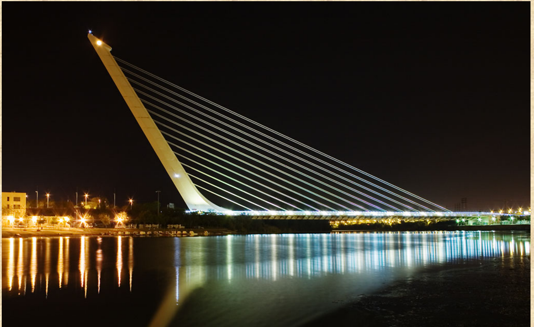
Seville - Alamillo Bridge - Santiago Calatrava - 1992 form: cable-stayed beam material: steel cables and reinforced concrete
